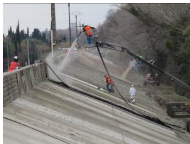
FIGURE 8 - PROJECTION DU BETON PROJETE (© COFEX MEDITERRANEE)
